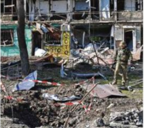
SHATTERED: A Ukrainian serviceman on Thursday was shot to an apartment building destroyed by shelling in Kramatorsk in eastern Ukraine. Russia intensified strikes on infrastructure, in particular in Ukraine's east, where some are fleeing into the country. AP
