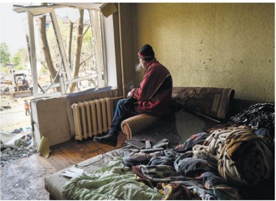
An airstrike blew out the wall of a home in Kramatorsk. A Ukrainian military official said that, remarkably, no one had been killed.
