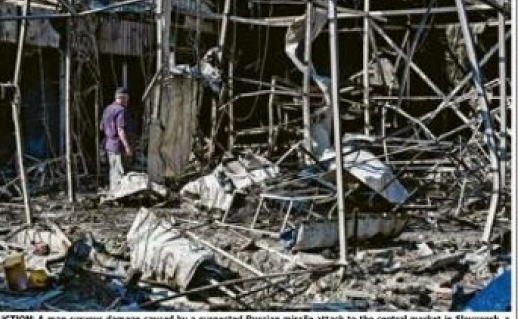
DESTRUCTION: A man surveys damage caused by a suspected Russian missile attack to the central market in Sloviansk, a city in Ukraine's eastern Donetsk region. A tactical shift by Russia is setting the stage for a protracted war of attrition.
